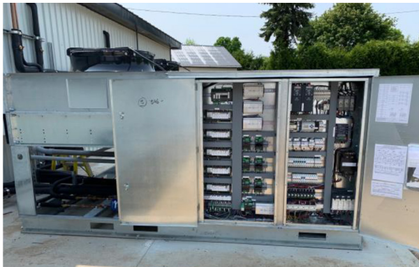
Figure 8. Post-project Arneg refrigeration case installation.
