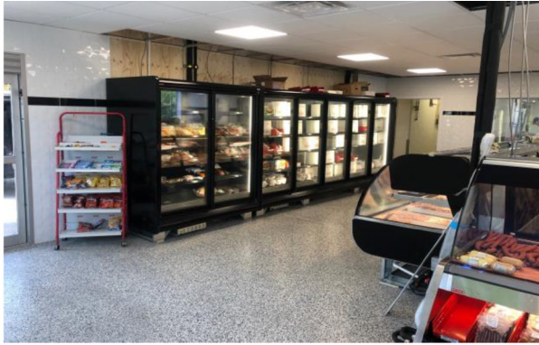
Figure 7. Post-project Arneg refrigeration case.
